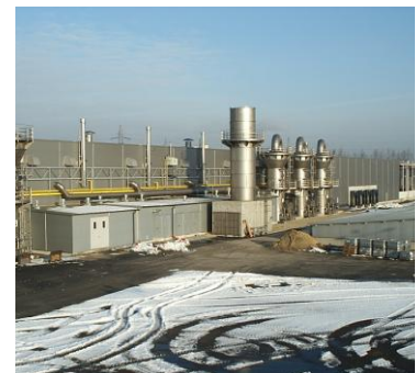
Scrubbers for oily fumes from aluminium die-casting machines
