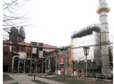
Filtration plant for cupola furnaces with CO oxidation, energy recovery (combustion air and hot water), SOx netralization, dedusting unit
